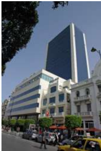
Ultra modern Hotel Afrique and old Colonial buildings side by side.
